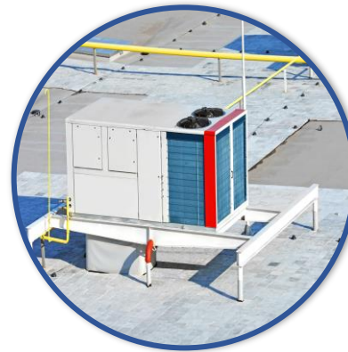
HVAC - Optimising & Coil Remediation
